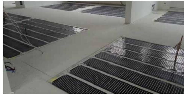
**SNOW CARPET** represents the ideal solution to avoid snow and ice setting in close to the buildings or on the roofs of the houses, deicing the pedestrian walks and the access ramps.
